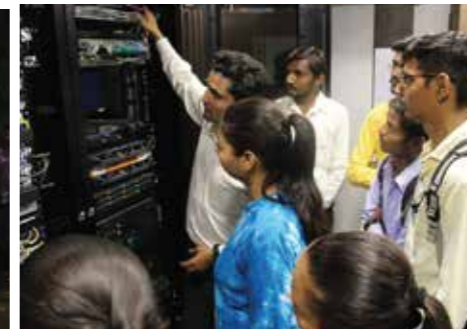
BSNL Ahmedabad Networking & Telecommunication server room
